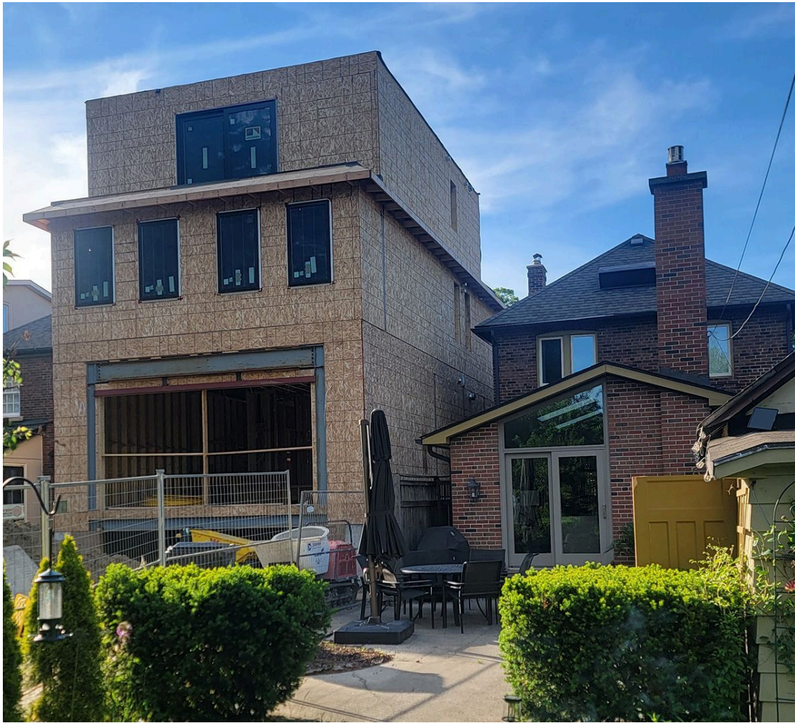
Rear of home under construction in the LPRO area which started out as a multiplex but will in fact be a 3-storey single family home.
