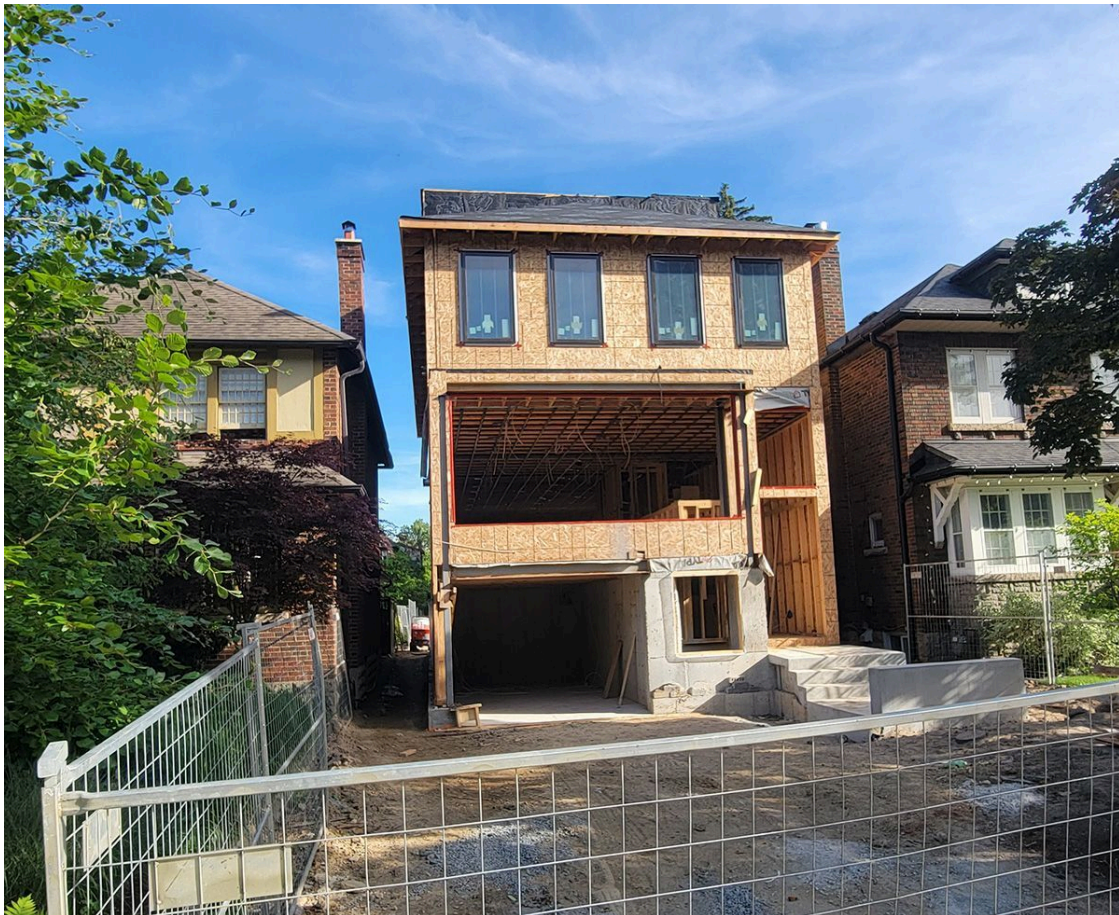
Front of home under construction in the LPRO area which started out as a multiplex but will in fact be a 3-storey single family home.
