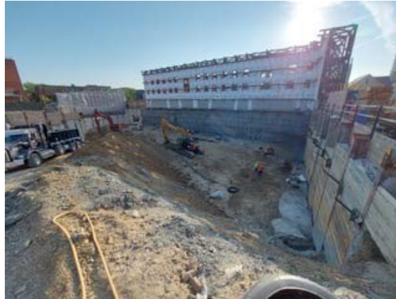
The excavation phase is almost complete!
